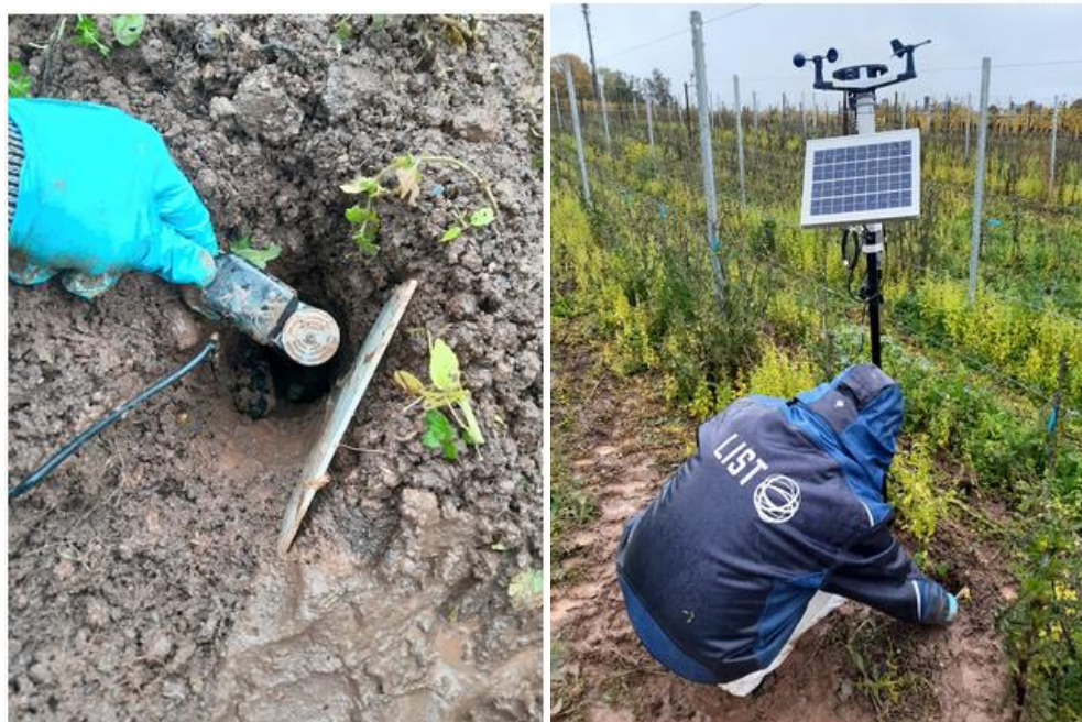
Figure 8 Installation of weather station, and soil moisture sensors in the LL1 (IVV Remich, Luxembourg)
