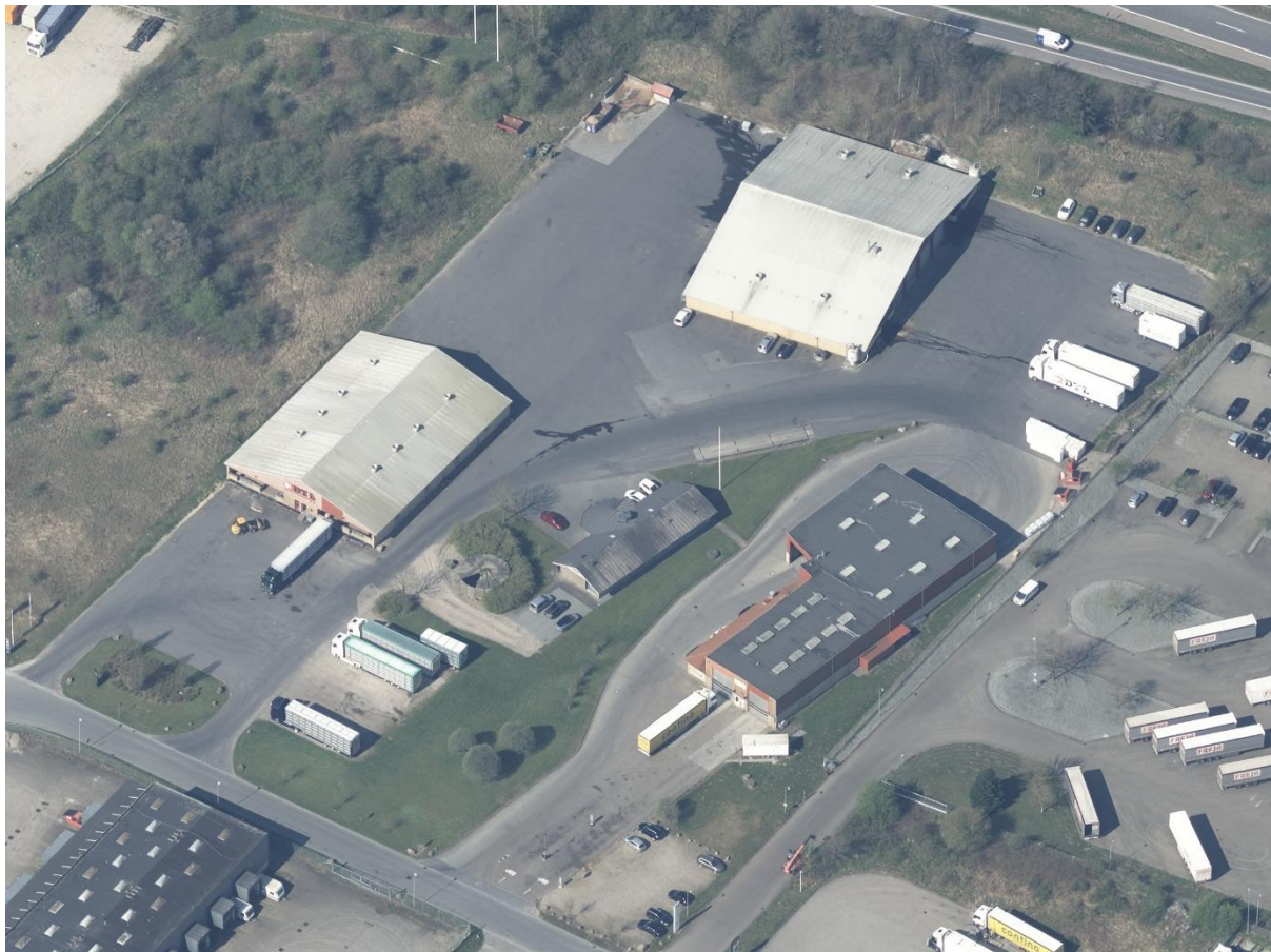
Figure 26 Orthophoto of the two DTL A/S assembly stables located at Industrivej 44, 6330 Padborg, Denmark (Dataforsyningen Skråfoto, The Danish Agency for Climate Data)
