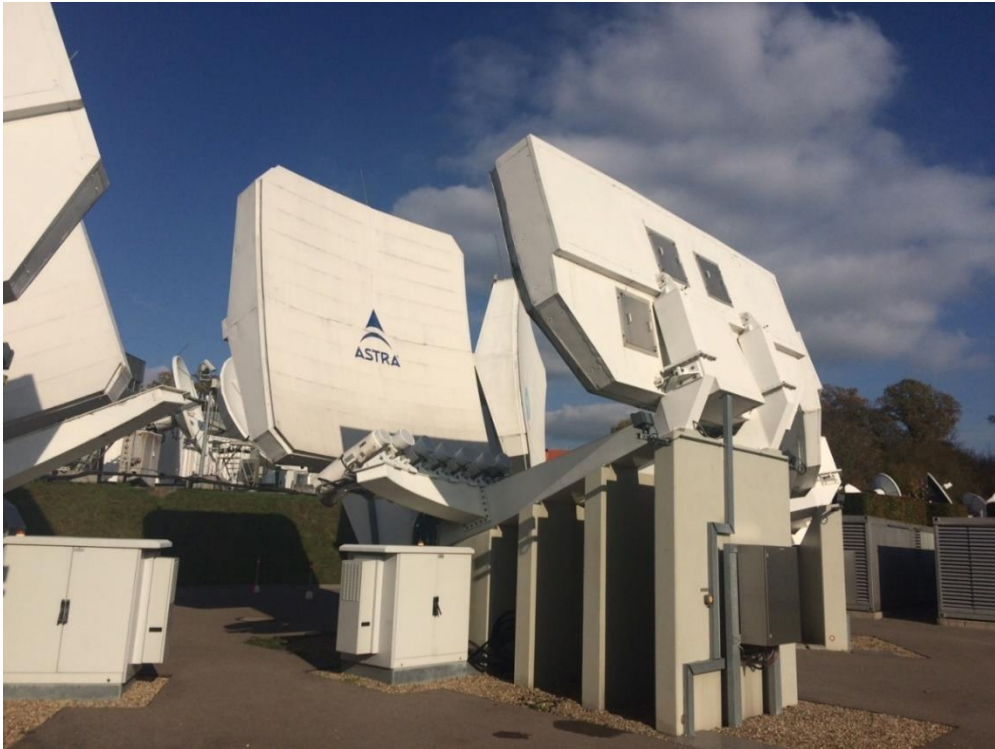
Figure 9: RF Downlink Ground Station: MBA#102 Antenna, Diameter: 4.5m, Multi-Beam Antenna, Rx only, Ku-band
