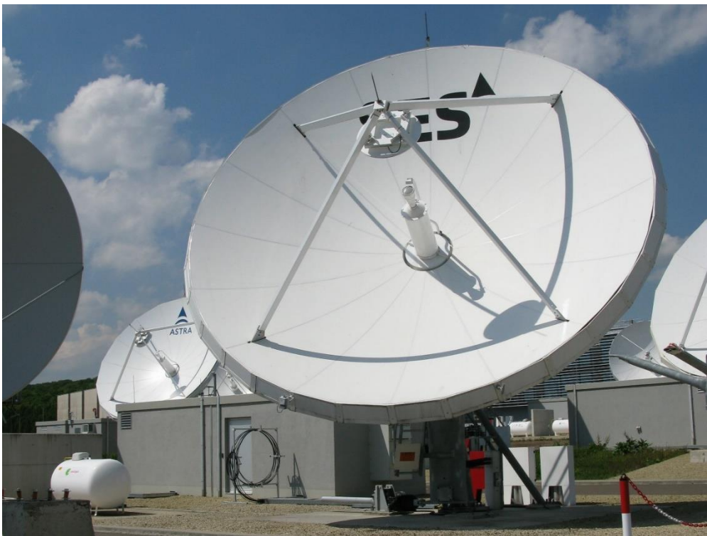
Figure 8: RF Uplink ground Station: ATF #33 Antenna, Diameter: 9m, Vertex, Tx/Rx, Ku-band
